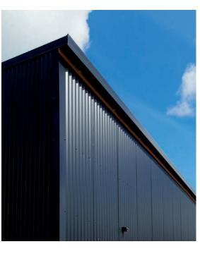
Technical: Armorsteel® ColorZen® conforms to AS/NZS2782:2013. Suitable for ISO9223:2012 Atmospheric Classifications C1 to C3, and for Roofing (not wall cladding) in C4. Refer to Armorsteel® Warranty & Maintenance Guide for full details.
